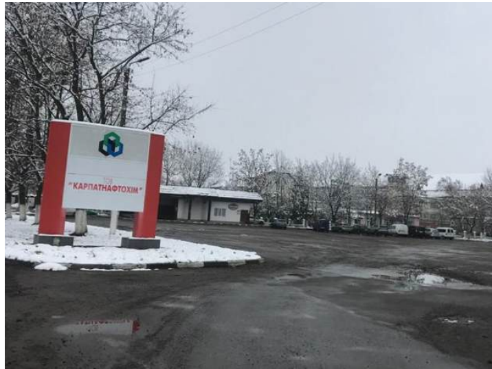
Karpatnaftokhim plant in Kalush, Ivano Frankivsk Oblast (ARMA/CC).
